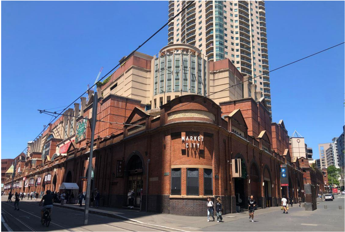
Figure 5: Site viewed from corner of Hay Street and Quay Street
