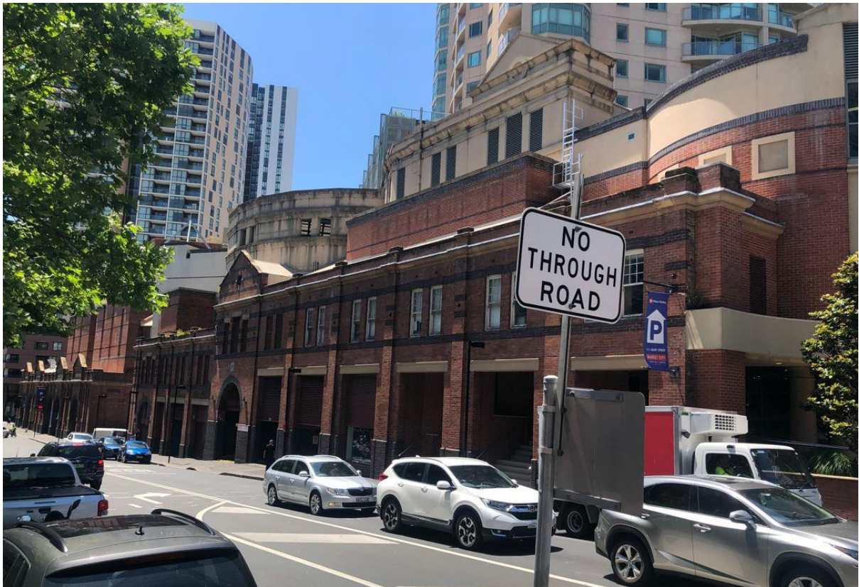
Figure 6: Site viewed from Quay Street looking north
